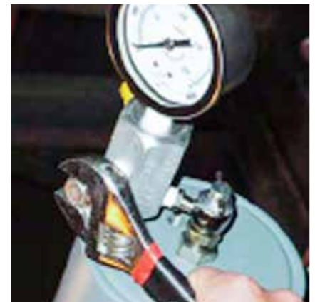
Gauge assembly affixed to gas valve—ready to bleed air from hose
