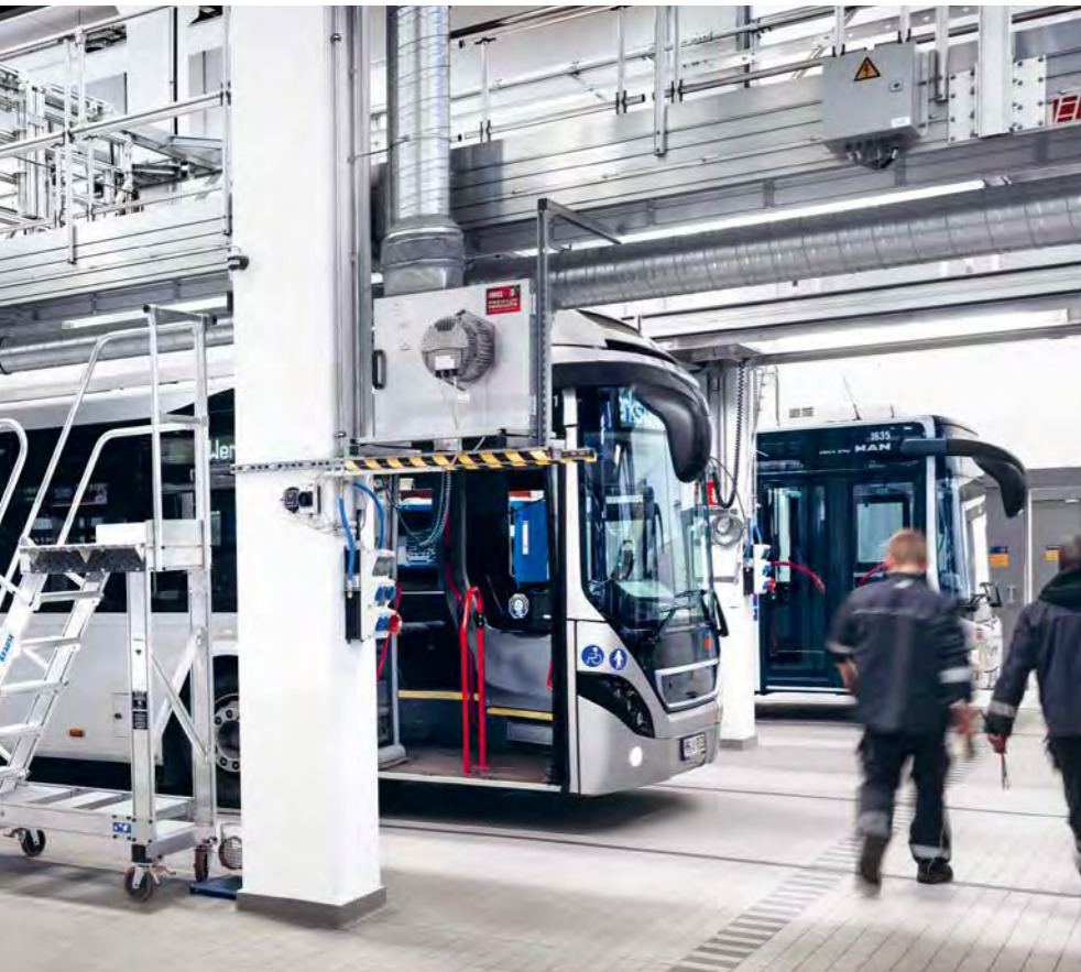
Building conversion: New plant space enables work on the roof.
